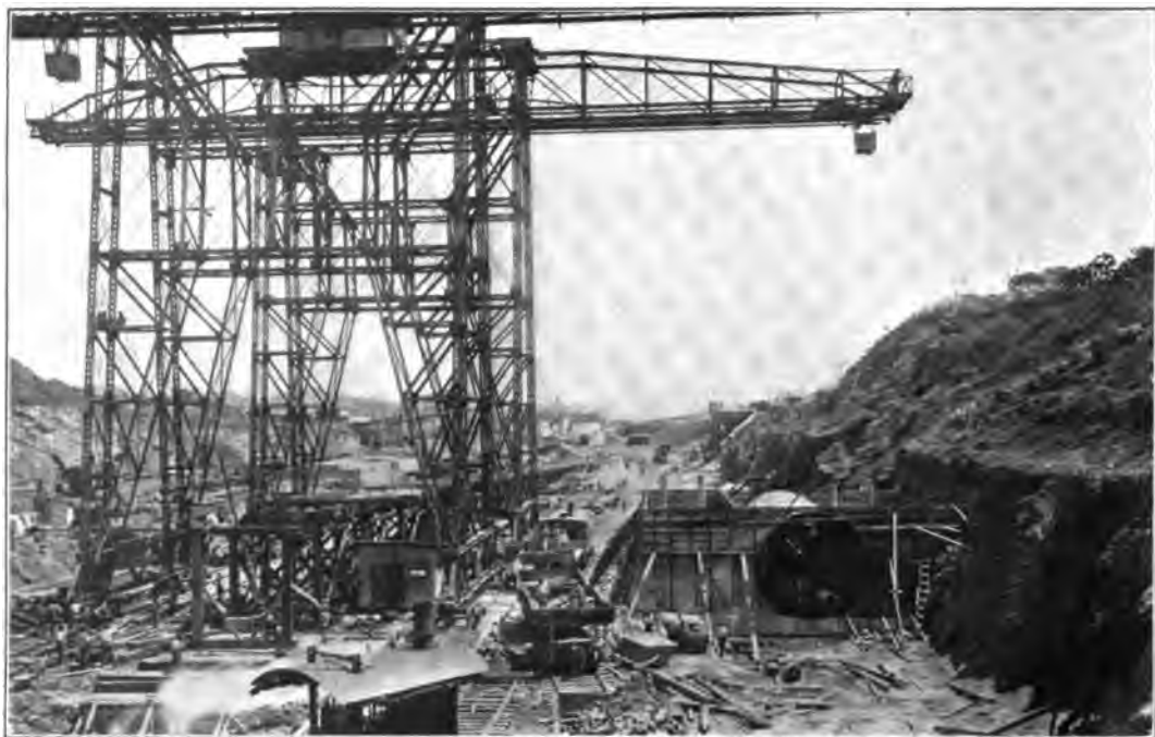
LAYING SIDEWALL CULVERTS, WEST CHAMBER, PEDRO MIGUEL LOCKS, MARCH 3, 1910.
